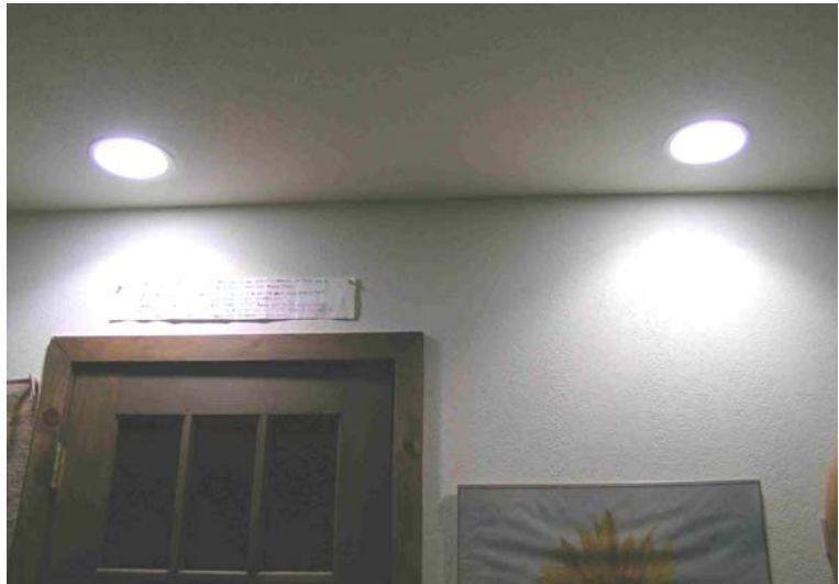
Figure 14. Light distribution with white reflectors and CFLs
