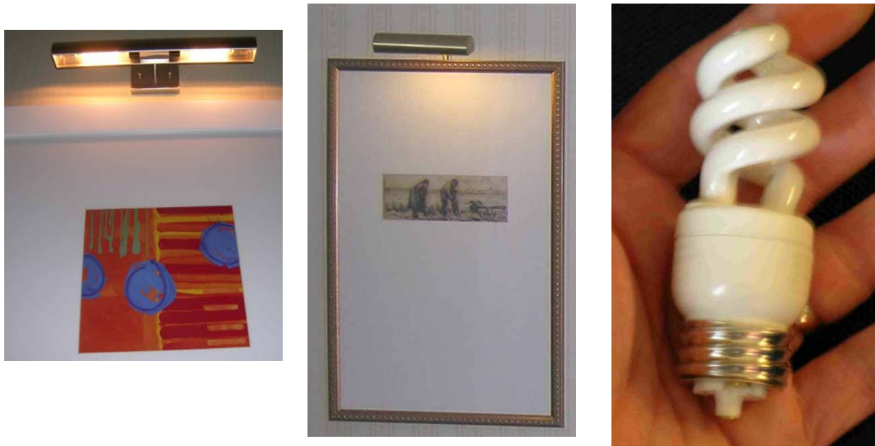
Figure 2. The painting on the left is illuminated by a pair of 20 watt incandescents while the one in the center by a pair of 4 watt CFLs, an example of which fits in the palm of a hand.
