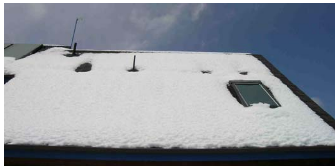
Figure 32. The two melted areas in the snow above the skylight correspond to recessed can lights that are almost never turned on. Melting is due only to air exfiltration from the conditioned space below the cans and the lack of insulation on top of them. The larger melted hole in the snow to the left of the vent pipe is due to a similar can above the shower which has a 250 watt infrared bulb in it. This light is on a timer and on average is illuminated about 12 minutes a day.
