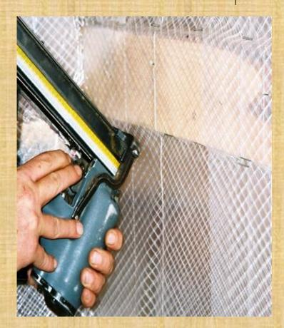
A small tube (1.5 inches od) is used to snake through a hole x'ed into the plastic. This ensures complete coverage with high-density cellulose. The result is excellent insulation and virtually no infiltration
